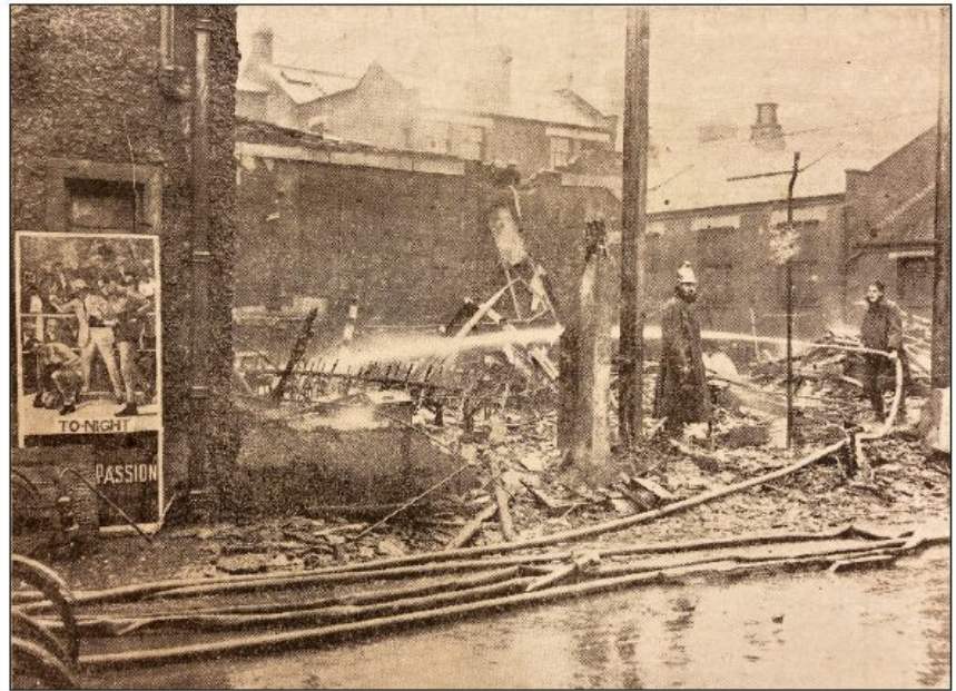
The end of the New Empire, 1926. Fire broke out in the early hours of Thursday 7 January, probably as a result of a cigarette dropped by a patron, following the final performance of Thorns of Passion – 'a thousand thrills in this mighty drama'. It was rather upstaged by reality; a poster advertising the evening's programme appears to be the only item to have survived.
